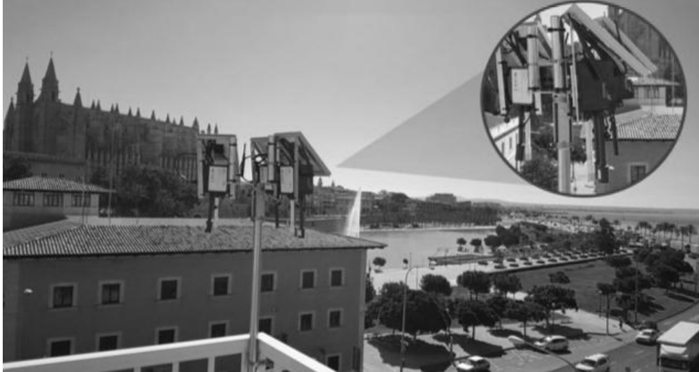
Figure 2. IoT Environmental Sensor installed at the Palma Port Authority Headquarters
