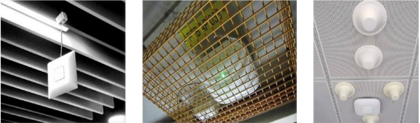
Figure 2: Examples of incorrect AP placement (courtesy of 7signals)
